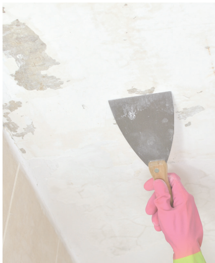
Removing chips
