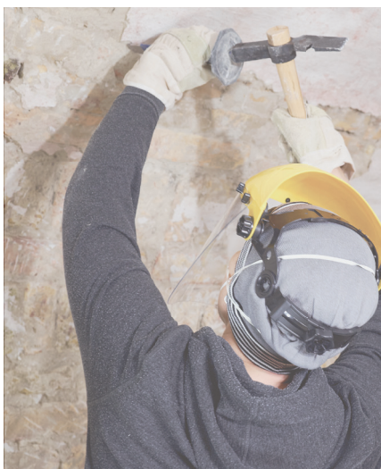
Chipping/removing layers or coating
