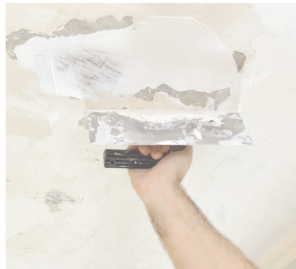
Crack Filling
