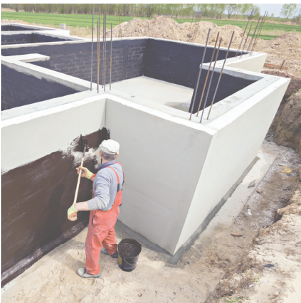
Exterior waterproofing with Brea (Pitch)
