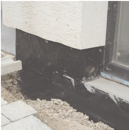
Exterior waterproofing with Brea (Pitch)
