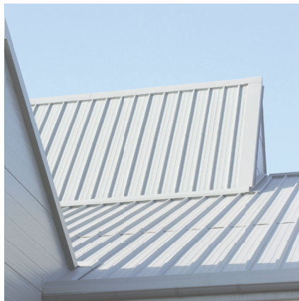
Insulating waterproofing the metal covering
