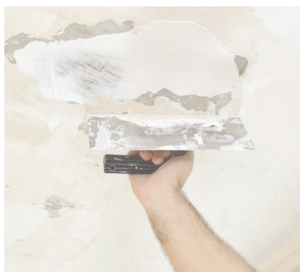
Crack Filling
