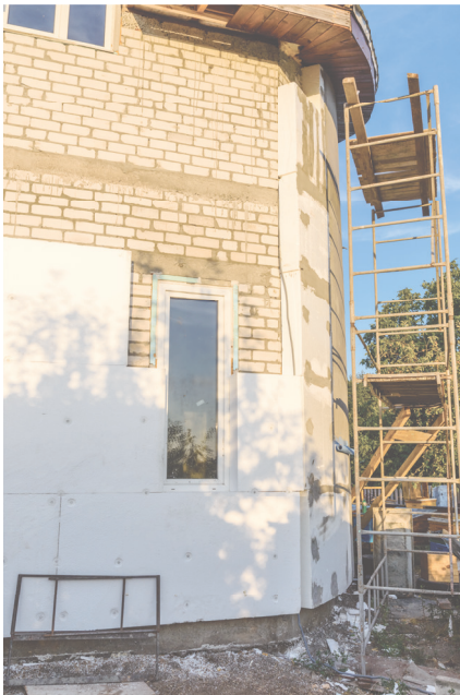
External Thermal Insulation System
