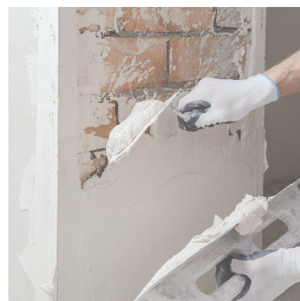
Re-coating with breathable plaster
