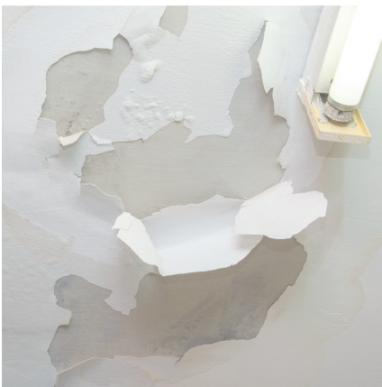
Damp through penetration/leak
