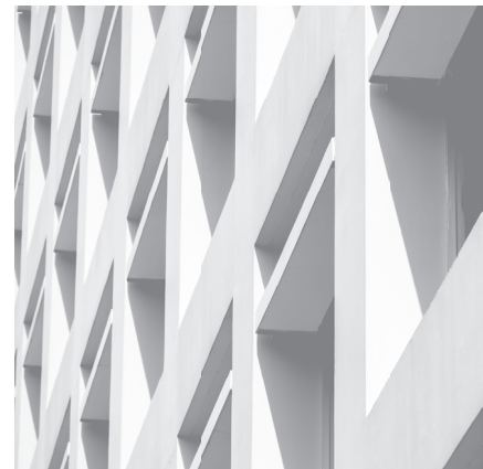
Waterproofing concrete and cement façades
