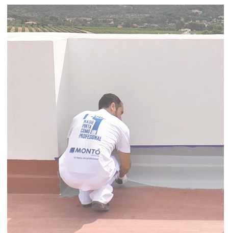
Reinforcing particular points
