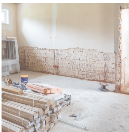
Wall exposed for evaporation
